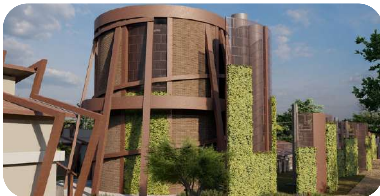
The HTMR-100 Kudu design. 50% of the reactor is under the ground.
