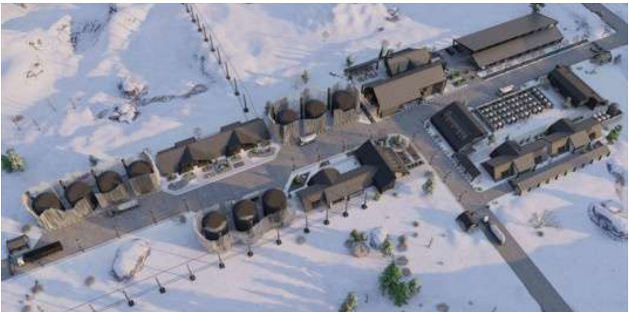
Sable Design of the South African HTMR-100 Small Modular Reactor. This is a 10-reactor setup that was developed as a result of a request from Lesotho. The request was for the reactors to be in a linear layout, so that it would fit on the side of a mountain, and also it had to be able to withstand snow. The architects are: JKDA Architects of Pretoria.
