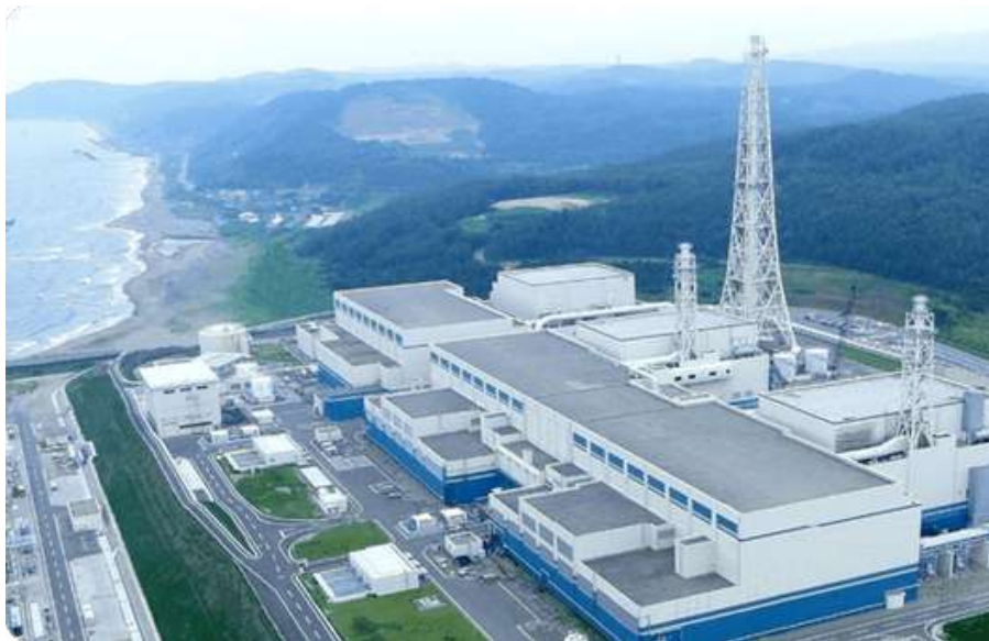
Picture: Kashiwazaki-Kariwa nuclear power station. Pic TEPCO
