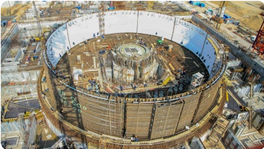
Unit II of Kursk II under construction.
