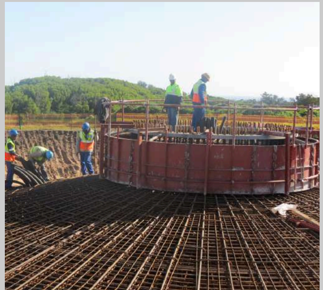
Wind Turbine Base - note the amount of steel!
