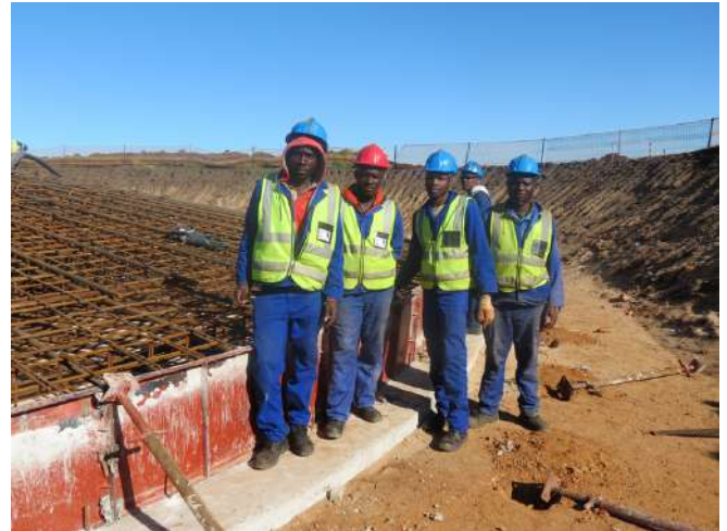
The work crew at the Wind Turbine base
