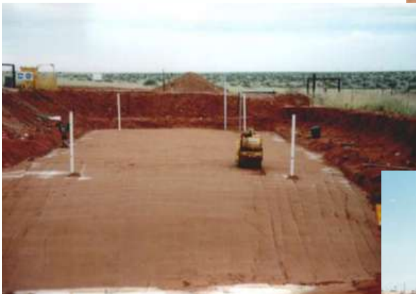
Capping of Disposal Trench
