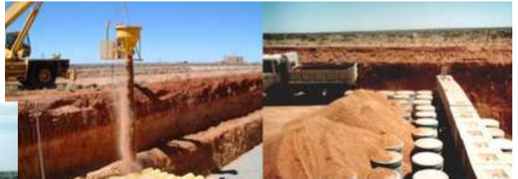
Backfilling of waste packages
