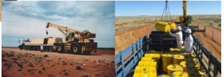
Disposal into trench
